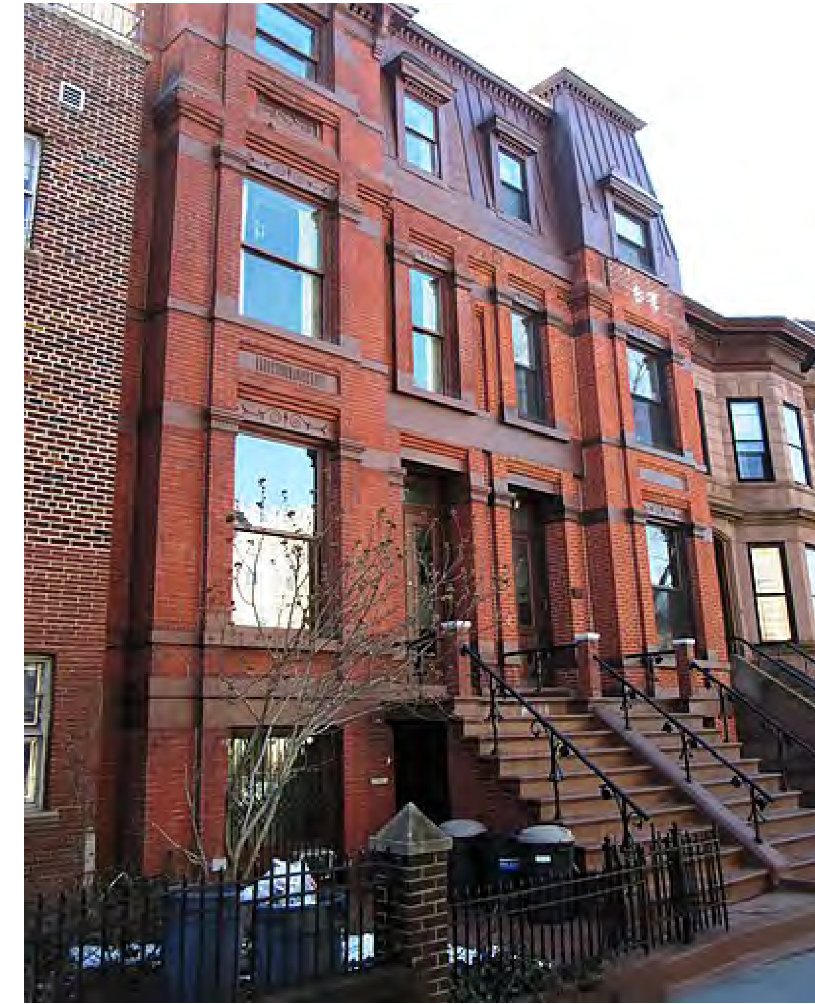
A brownstone building with waste and recycling bins set out front
