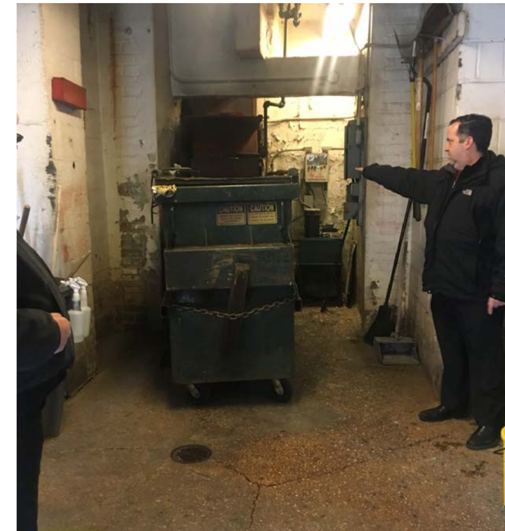
A visit to a building's trash room.
