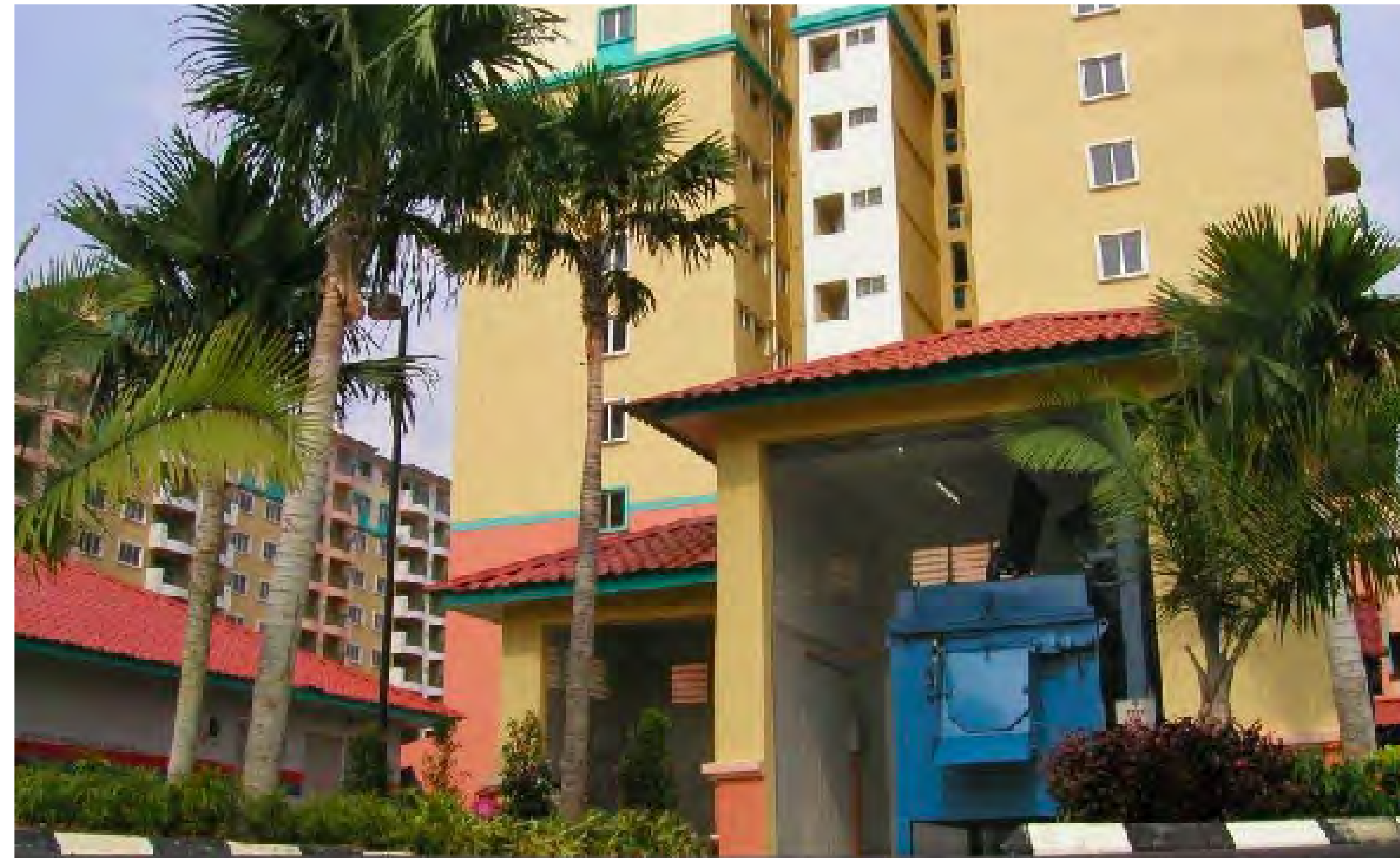
Above: Pneumatic Waste Conveyance System (PWCS) collection bins at a residential development in the SSTECC.
