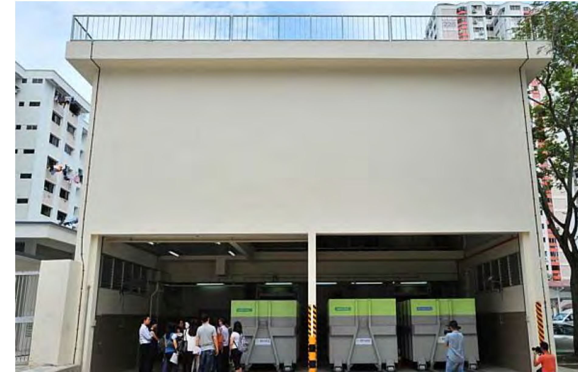
Centralised pneumatic waste bin center with roll-on roll-off containers.
