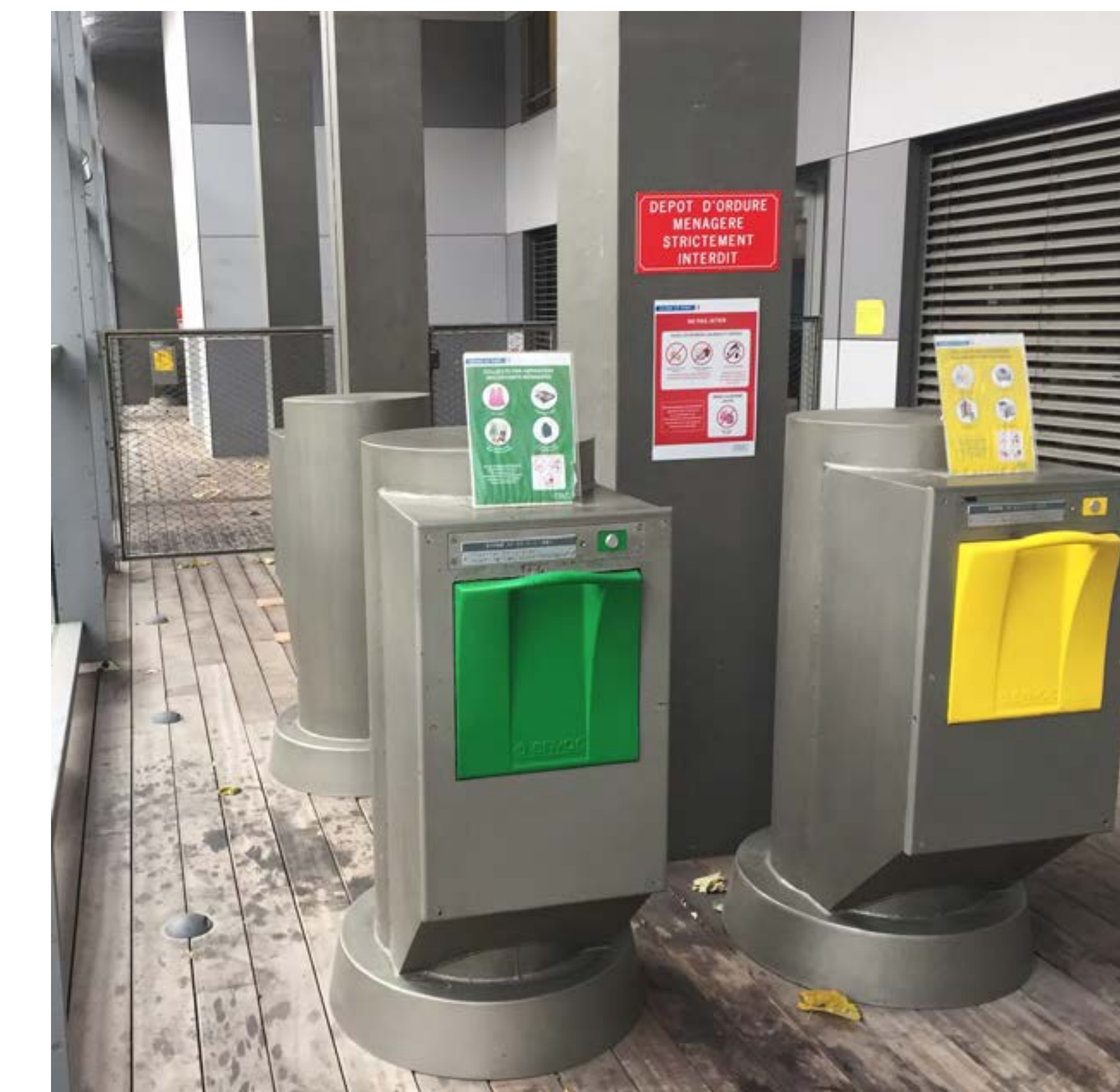
Residents bring waste down to the building lobby area and pneumatic tubes transport waste directly to the centralized containers in Paris, France.
