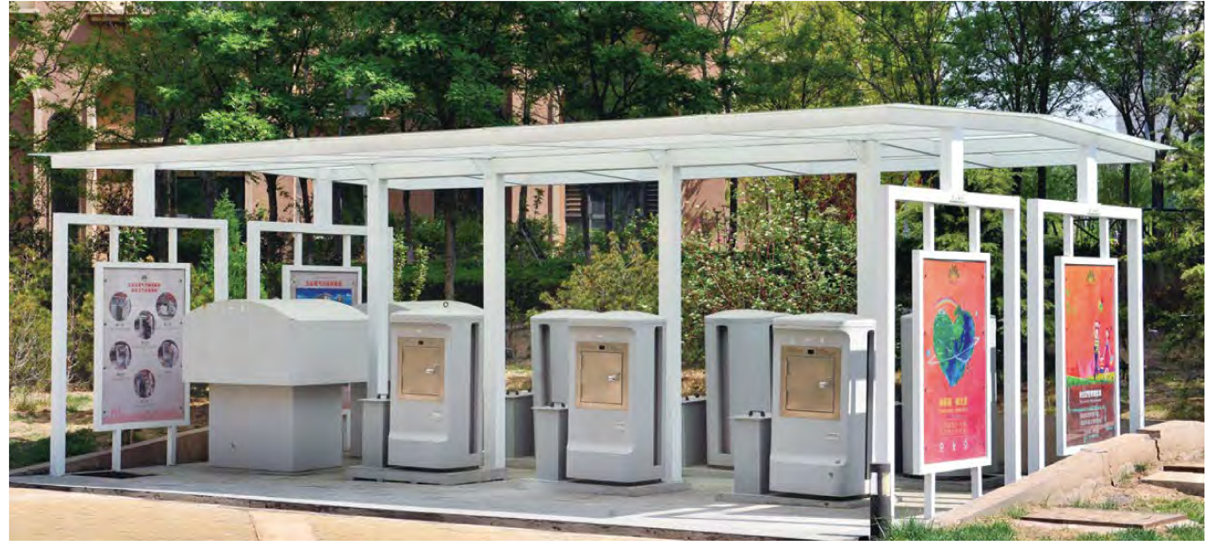
Above: Pneumatic Waste Conveyance System (PWCS) collection bins at a residential development in the SSTECC.
