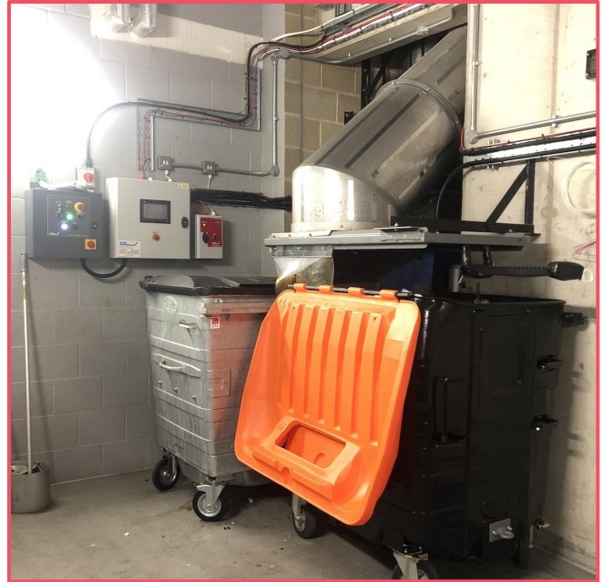
Chute compactors in London and elsewhere feed directly into wheeled bins. System shown above in London, by Hardall, see case study . NYC’s existing chute compactors can be retrofitted to feed into the same type of bins.
